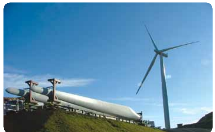
Meridian Energy's West Wind wind farm, to the west of Wellington, was fully commissioned in October 2009. It generated 497 gigawatt hours (GWh) in the year to 30 June 2010.
